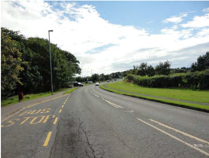
Culmore Road - View back towards Derry direction
