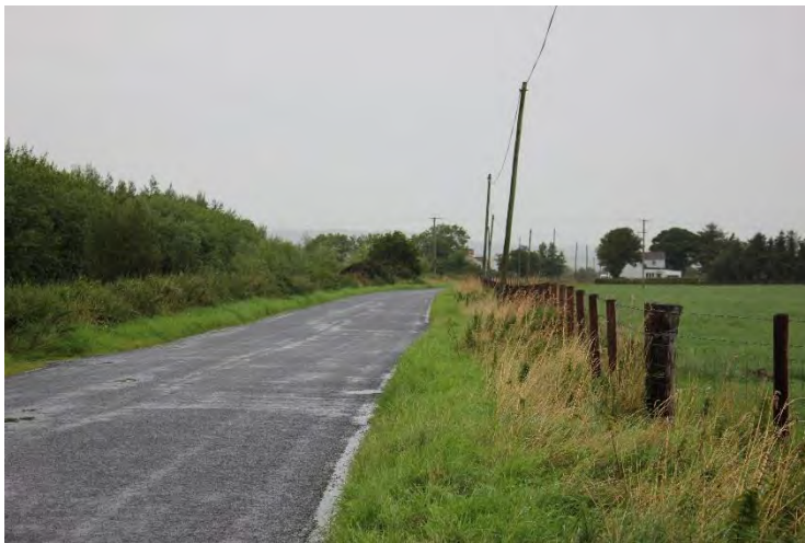
View north along Coney Road.
