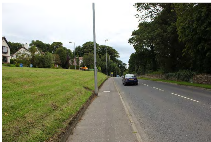
View north along A2 Culmore Road at Larcom Drive.
